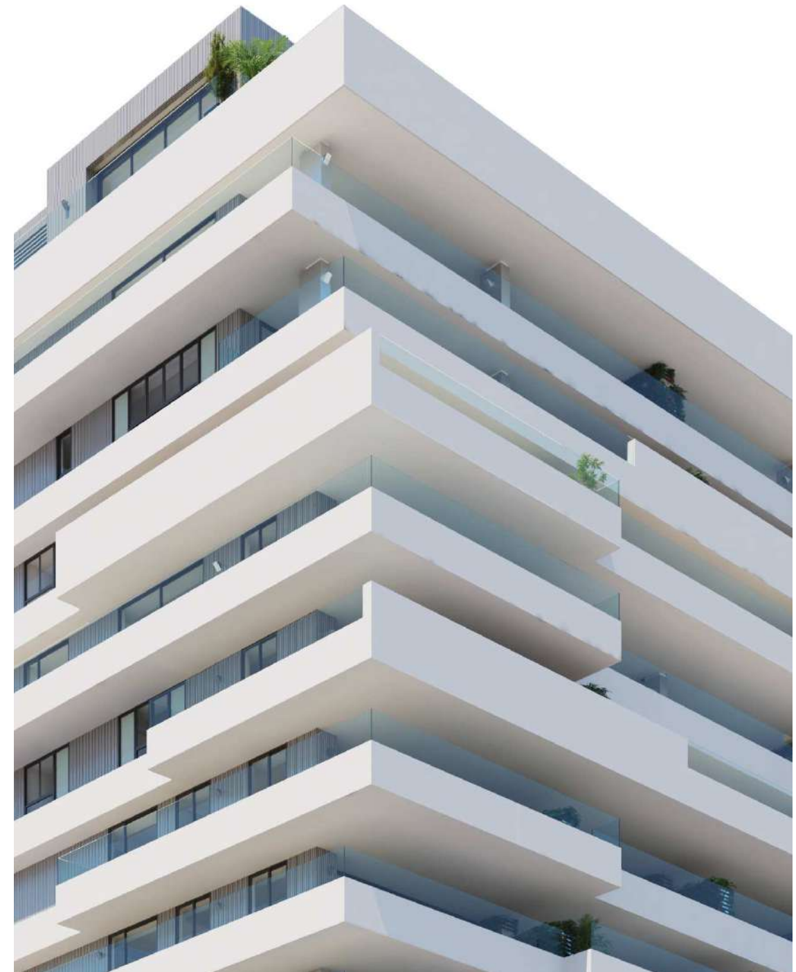
THE PARAPETS ARE MADE OF DOUBLE-SKIN FACADES WITH SOLID SURFACE OR CERAMIC PANELS WHICH ARE MECHANICALLY ANCHORED TO THE FLOOR SLABS
