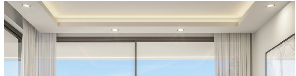
LED spot light & cove lighting
